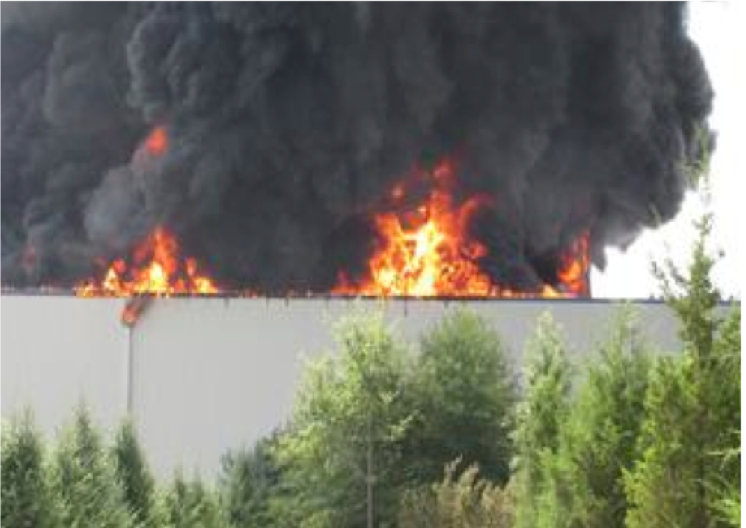
Fig. 1. PV roof fire at a refrigerated warehouse in NJ in 2013 (photo courtesy of Vince Lattanzio, NBC Philadelphia)
